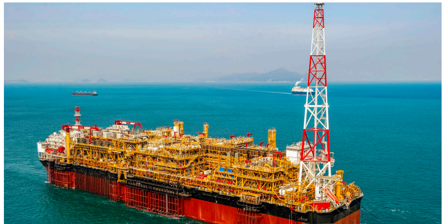
Corrosion Under Insulation
